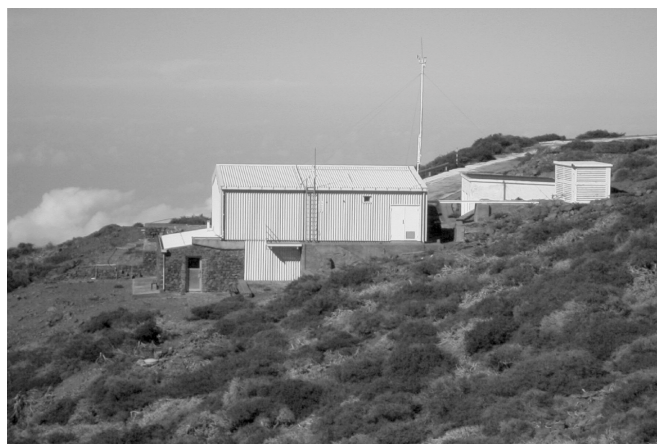
Fig. 2. The CMT building. Below the main structure can be seen the observers flat where the observer (when present) would sleep during the observations. On clear nights, the left side of the upper building slides out over the flat so that the telescope can observe.
