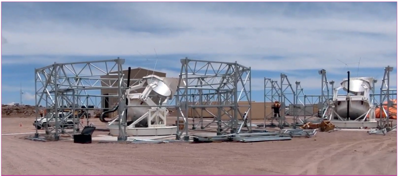
Fig. 1: Two of the three SATs, and their associated ground screens, on site in Chile. SO:UK will add a further two SATs and Japanese colleagues will provide a further one, totalling six.
